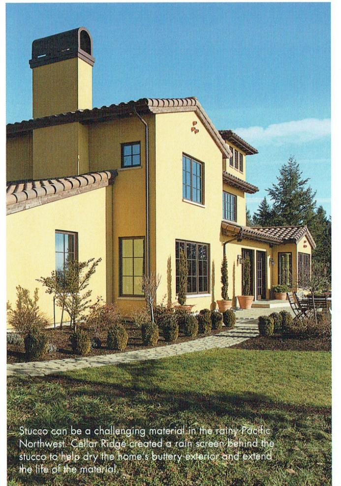
Stucco can be a challenging material in the rainy Pacific Northwest. Cellar Ridge created a rain screen behind the stucco to help dry the home's buttery exterior and extend the life of the material.
